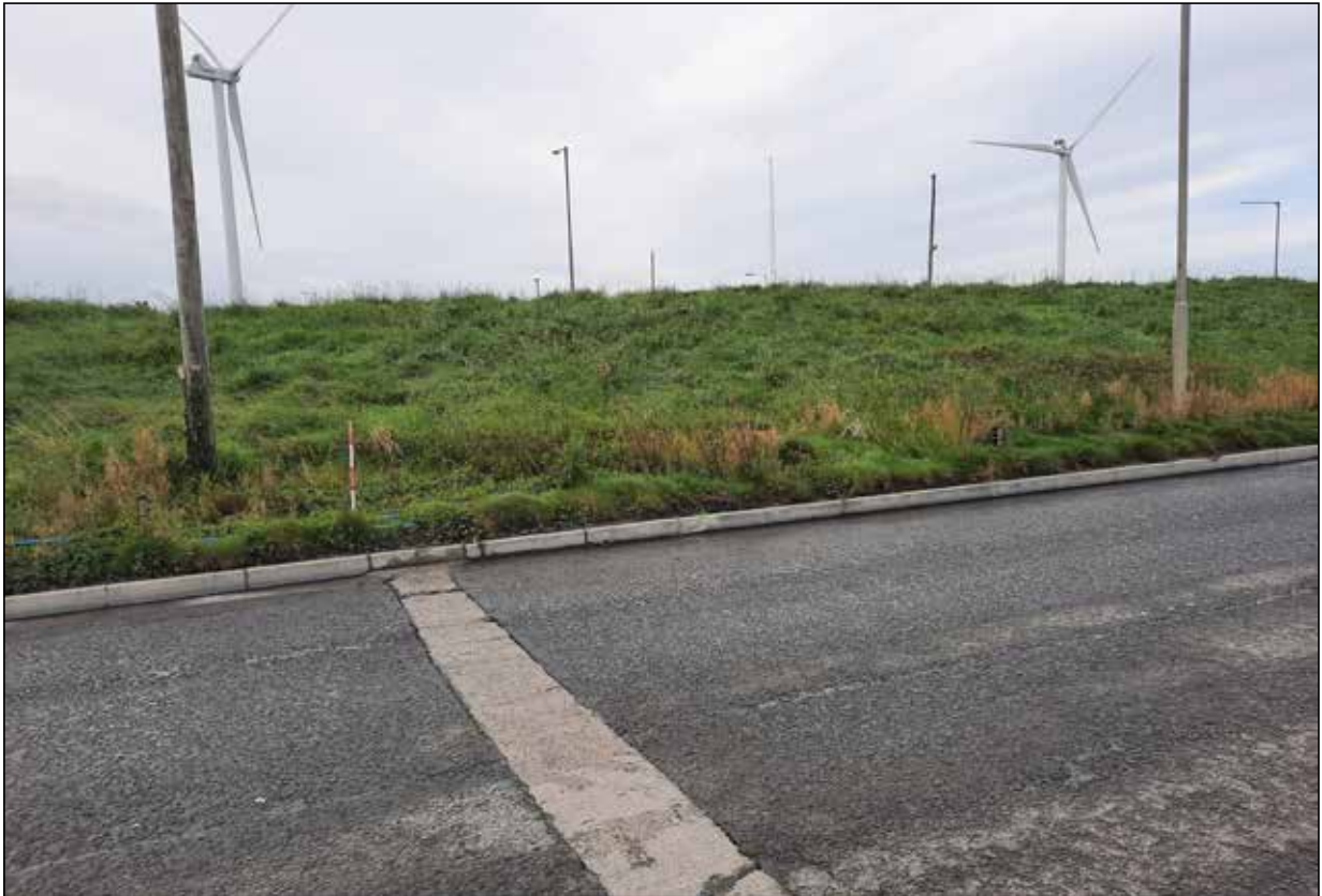
Plate 3 - Location of CH025 (stream, possibly culverted), facing SW
