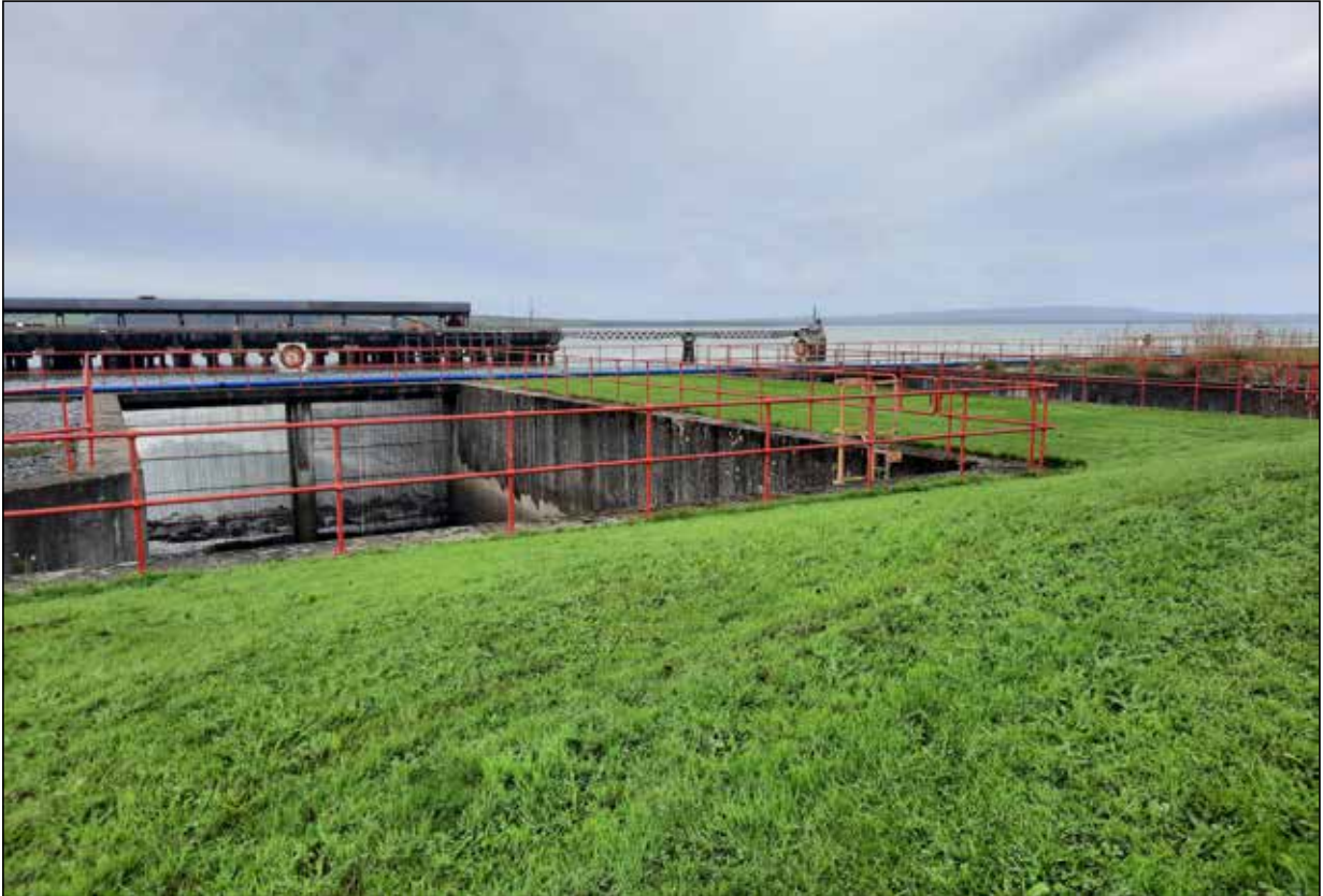
Plate 1 - View of Location of CH031 (Salmon Weir), facing SW
