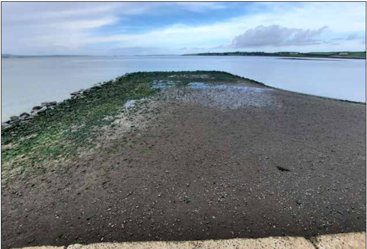
Plate 4 - View of CH021 (Jetty), facing W
