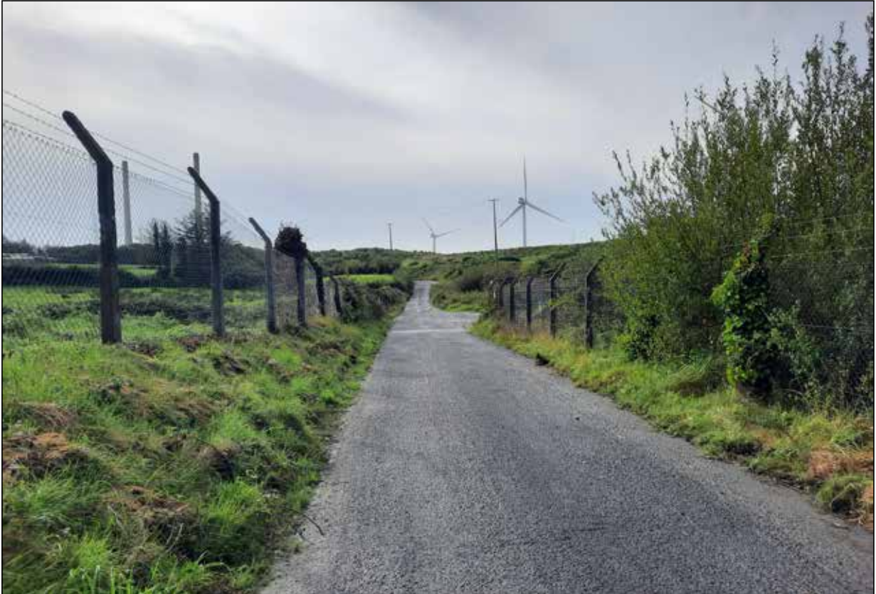
Plate 17 - View of Access Road, facing SE
