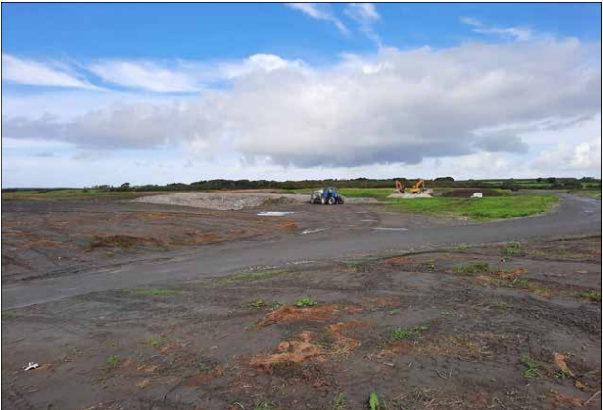
Plate 18 - View of eastern portion of Ash Storage Area, facing NE
