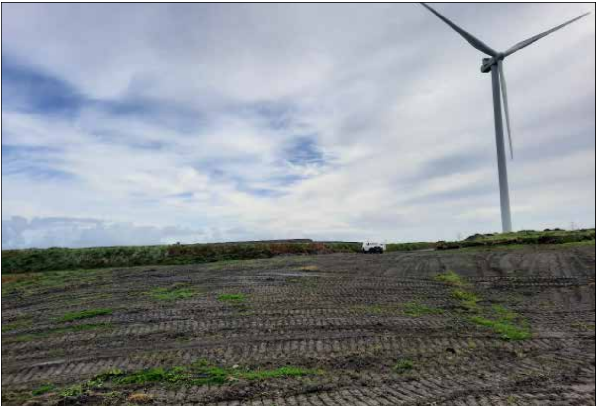
Plate 8 - Overview of southern portion of Ash Storage Area, facing N
